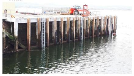
The harbour showing off its new greenheart fenders and just visible top left, the start of the new sheds.
